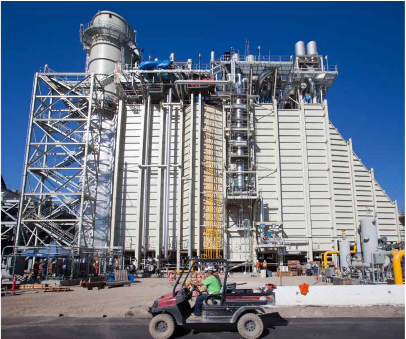
**Once-through HRSG.** Nooter Eriksen three-pressure heat recovery steam generator with Benson once-through technology equipped with SCR and CO catalyst to minimize emissions.
