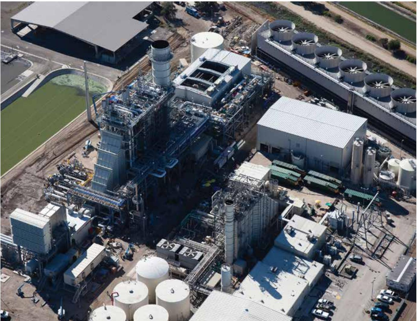
**Lodi Flex 30 project.** First operating Siemens Flex 30 combined cycle gas turbine power plant in the United States is nominally rated at 300MW net plant output and 57.8% net efficiency.
